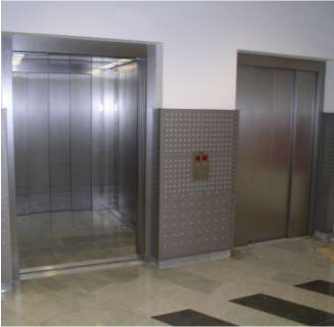
Above: 1000 kg MRL passenger lift for restaurant and airport terrace Left: two 1600 kg MRL elevators for parking house of the airport
