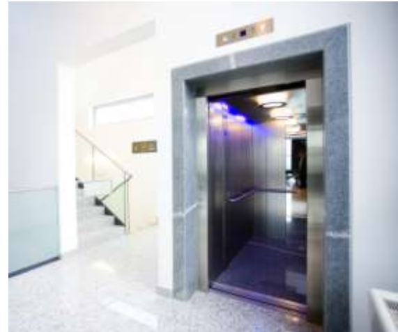
Above: 1000 kg MRL passenger lift for restaurant and airport terrace Left: two 1600 kg MRL elevators for parking house of the airport
