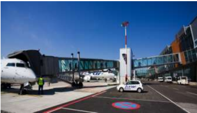
Above: 4 pcs boarding bridges for Terminal 1 Right: panoramic elevator and escalator for „Departures/Arrivals“
